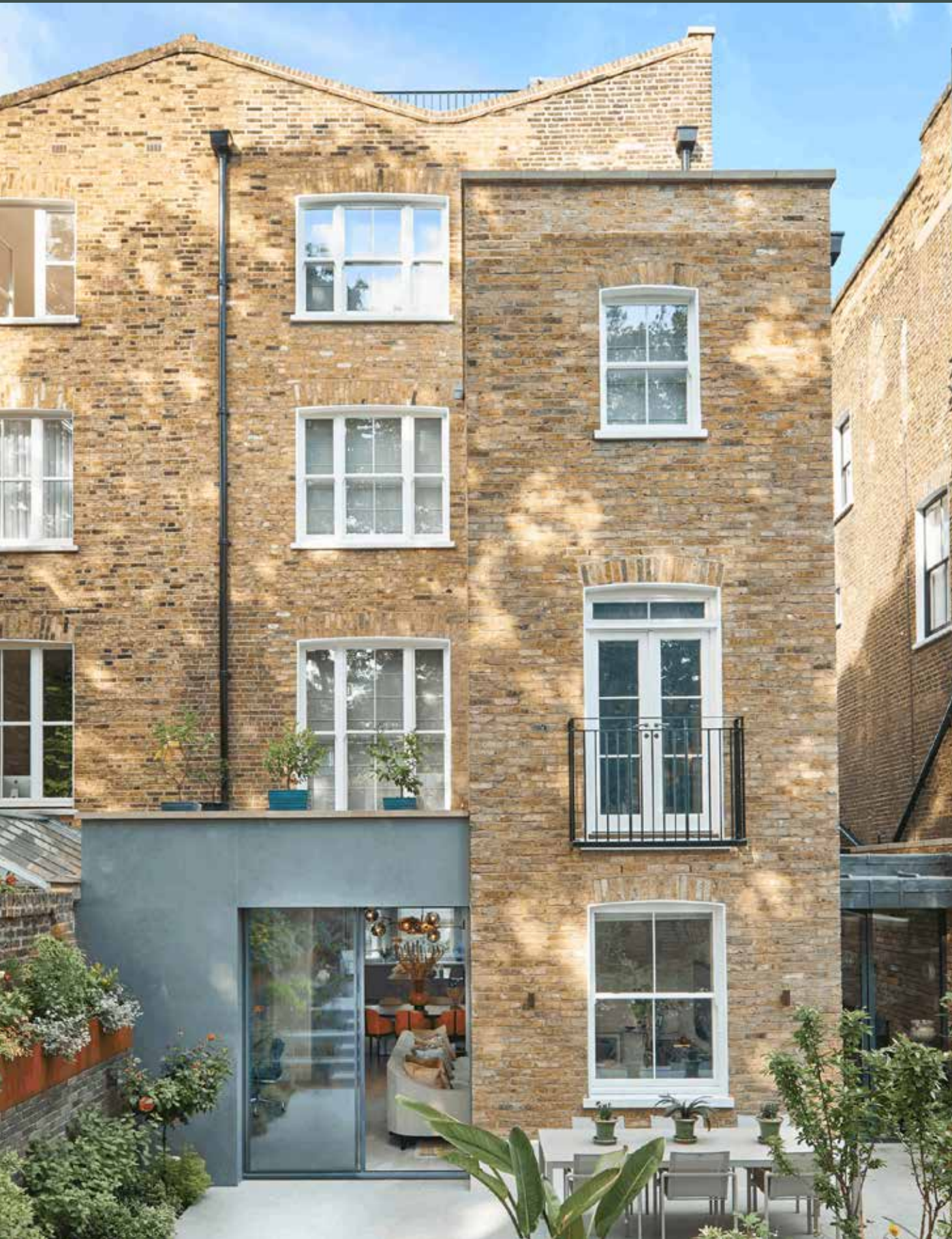
(HERITAGE TIMBER SASH WINDOWS AND FRENCH DOORS)
