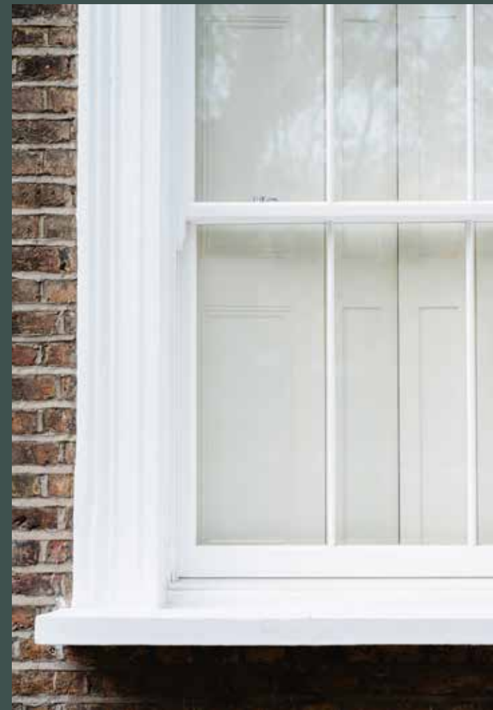
(VICTORIAN TIMBER SASH WINDOW)
