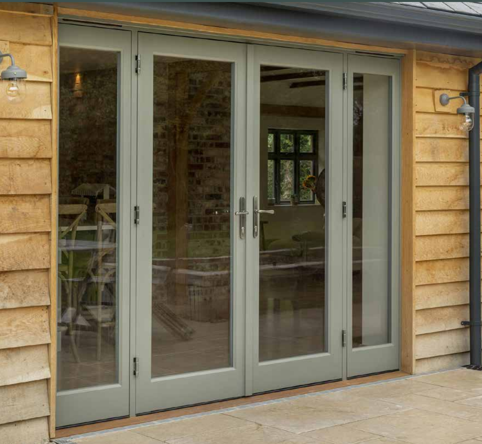
(TIMBER FRENCH DOORS IN BARN CONVERSION HOUSE)
