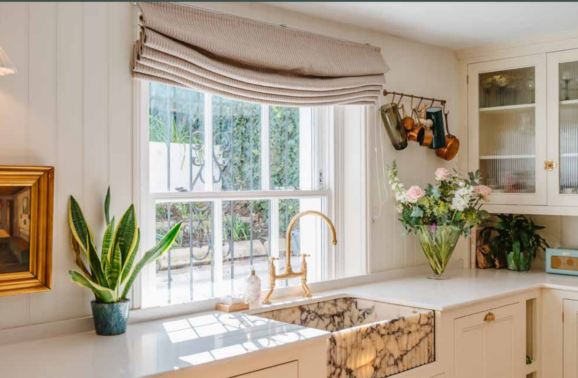
(TIMBER SASH WINDOW WITH ASTRAGAL BARS)
