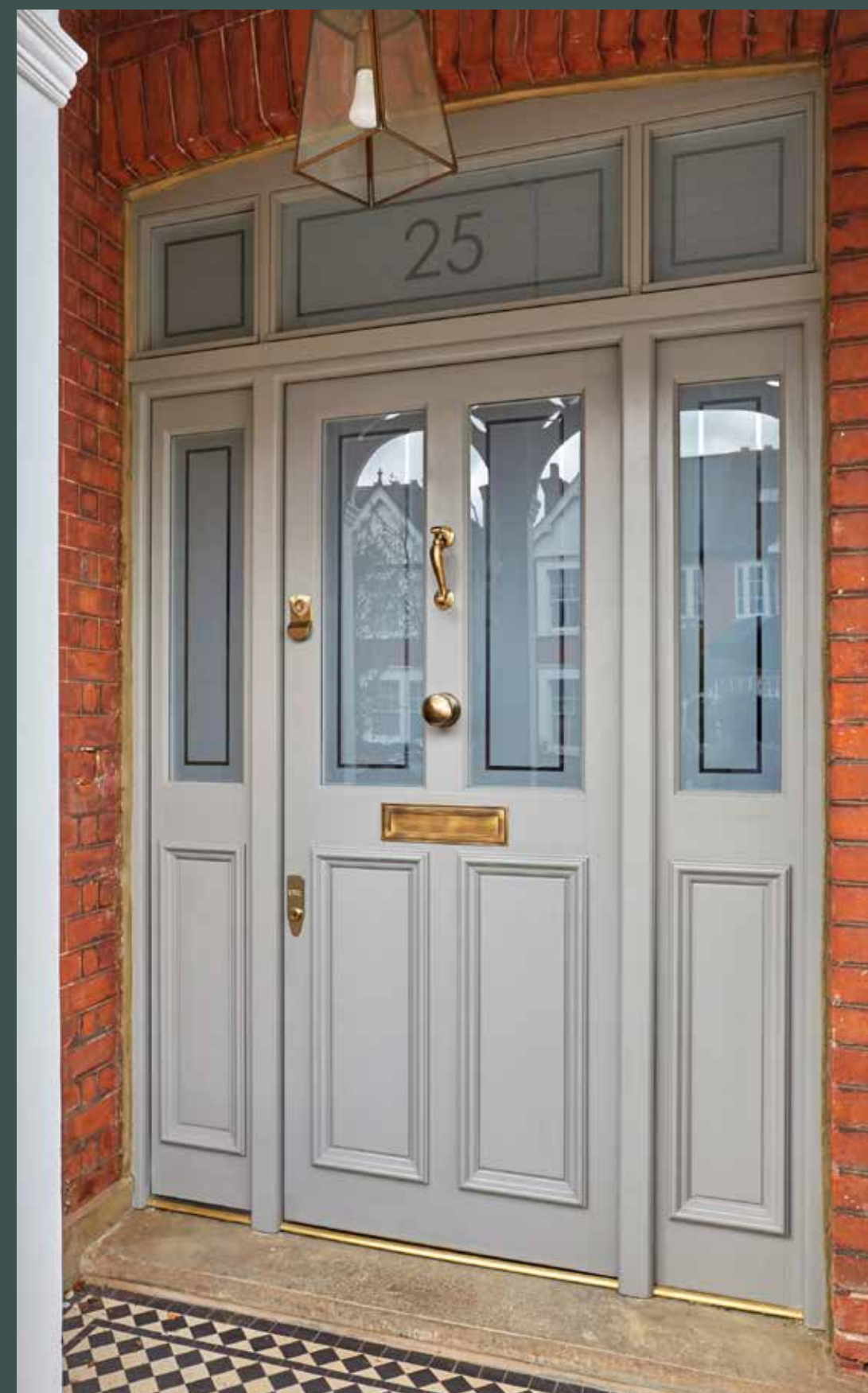
(VICTORIAN ENTRANCE DOOR WITH BOLECTION MOLDS & BANHAM LOCKS)
