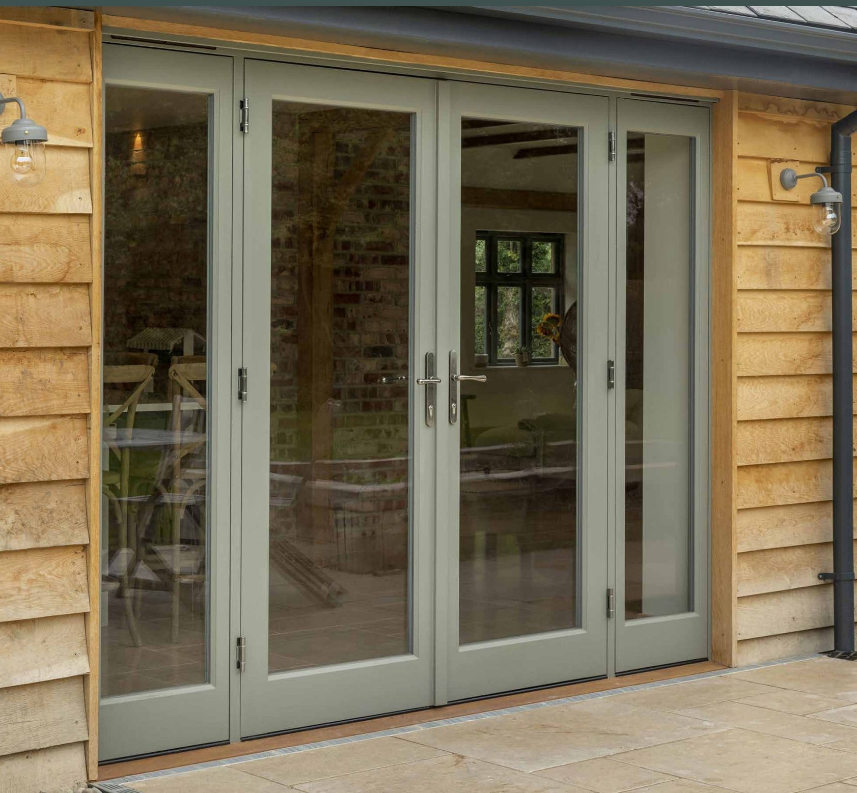
(TIMBER FRENCH DOORS IN BARN CONVERSION HOUSE)
