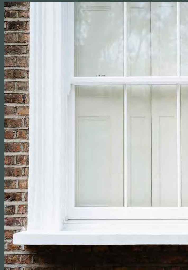
(VICTORIAN TIMBER SASH WINDOW)
