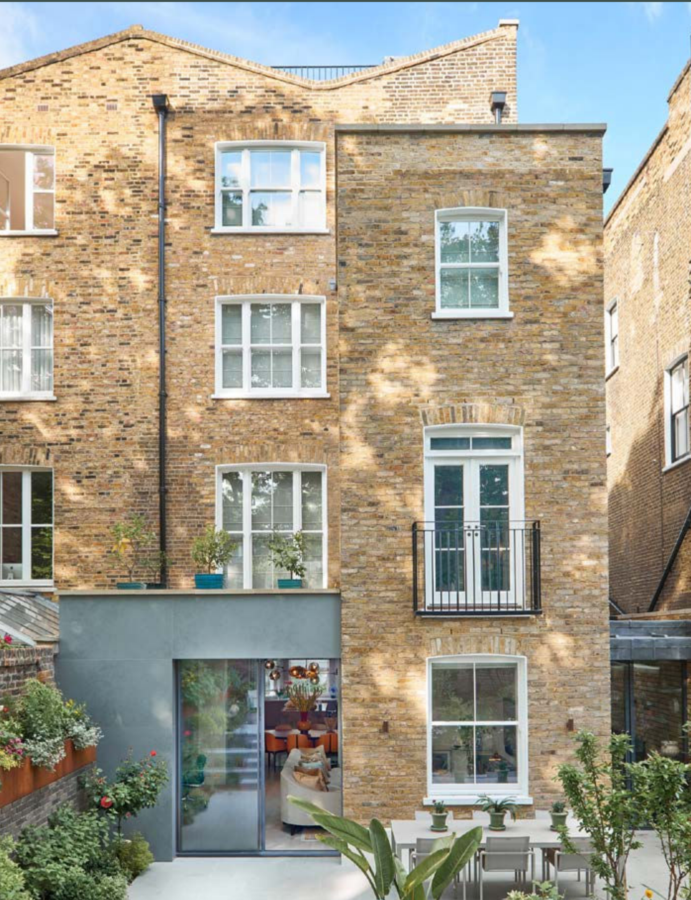
(HERITAGE TIMBER SASH WINDOWS AND FRENCH DOORS)
