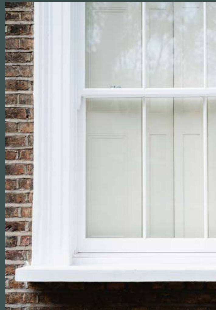
(VICTORIAN TIMBER SASH WINDOW)
