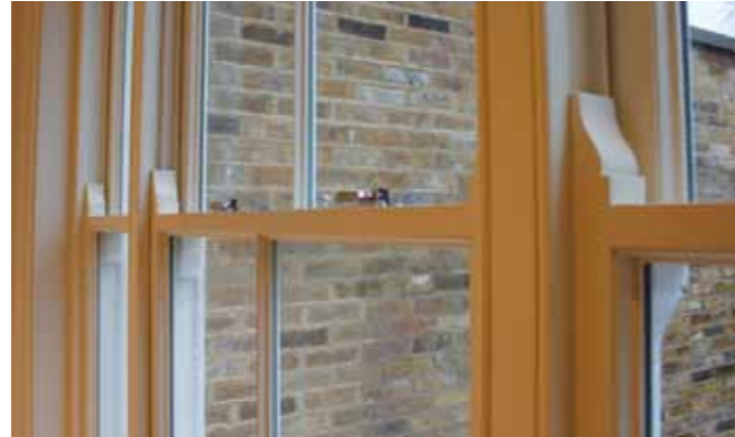
HERITAGE TIMBER DETAIL
